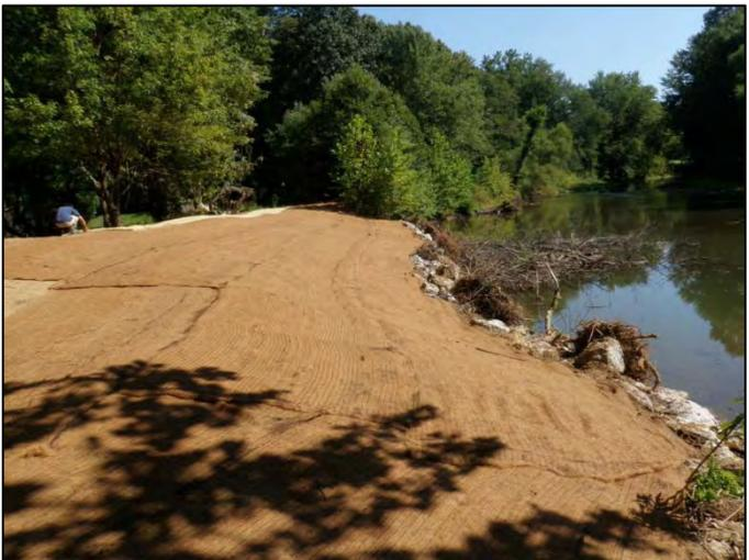
A Bobcat 337 Excavator (shown above left) and Bobcat T300 Track Loader were used to construct the project. A double net coconut coir erosion control blanket was used to provide immediate stabilization of the banks.
