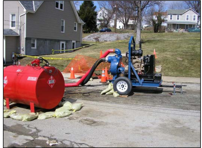
6" pump at "blowout" on Liberty Street. EIS began pumping on March 2, 2005.
