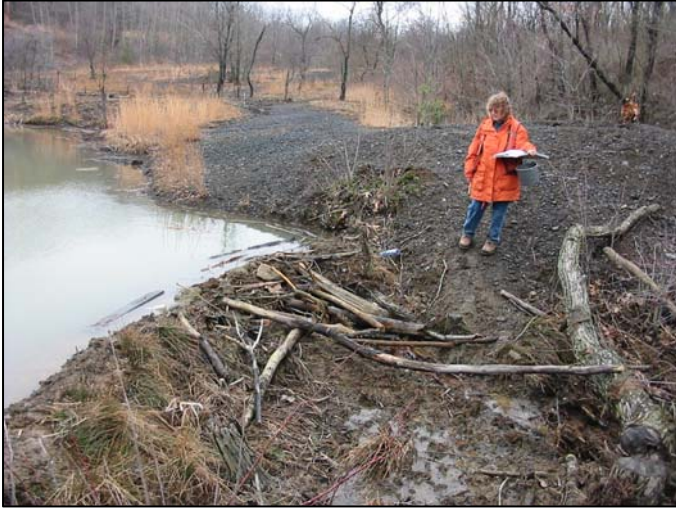
Inspections conducted to determine site conditions. (March 28, 2005)
