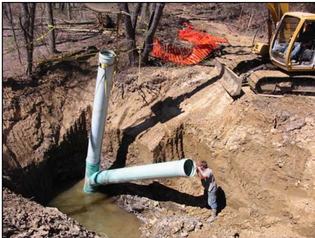
Installation of riser with custom perforations and overflow pipe. (April 13, 2005)
