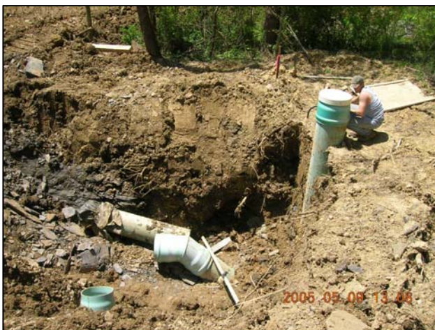
Elbow attached for piping to convey overflow to outlet channel. (May 9, 2005)
