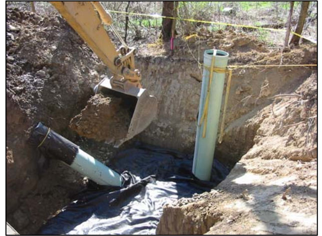
Geotextile used for layer separation of aggregate and backfill material. (April 13, 2005)
